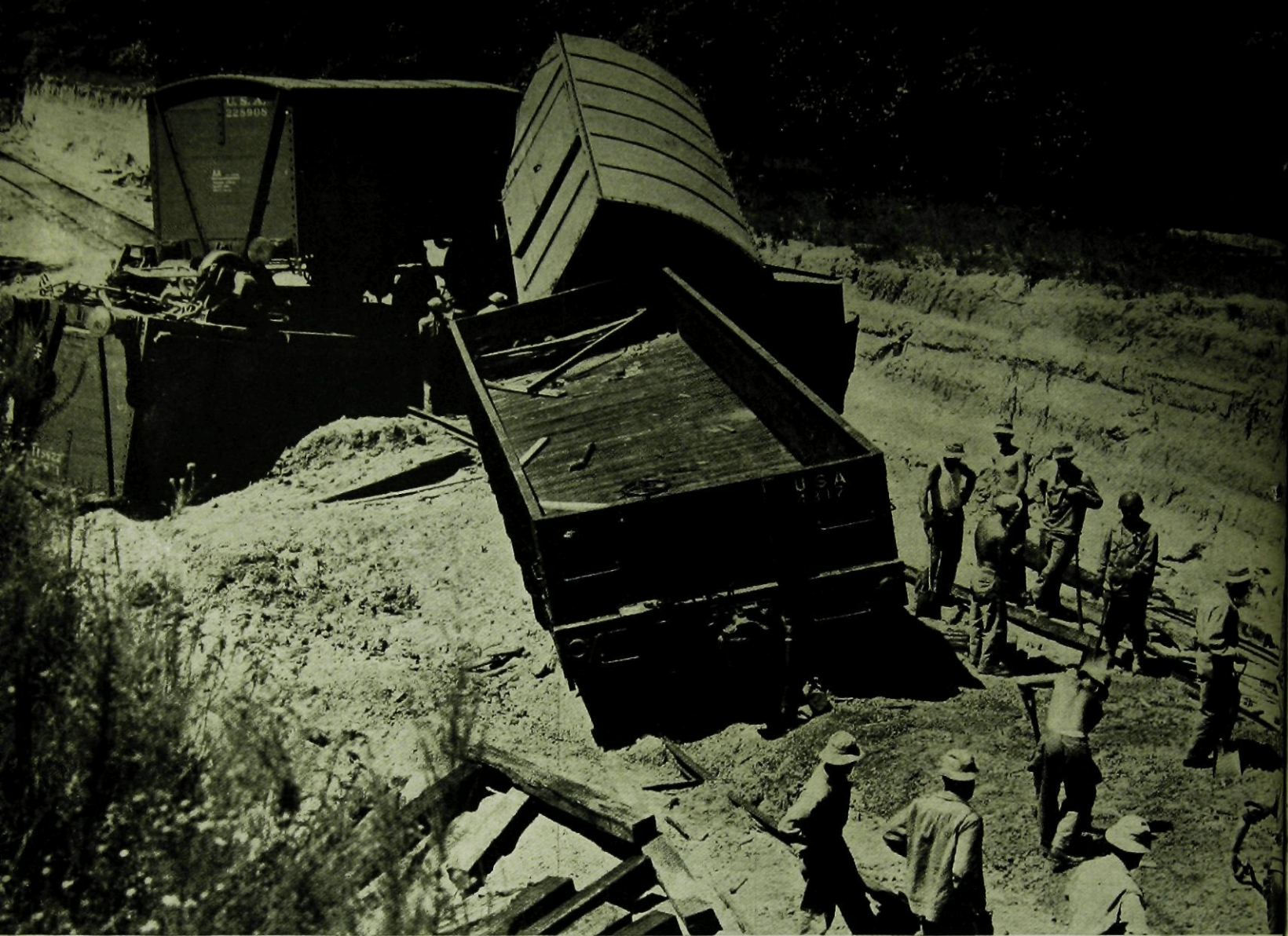
The Claiborne and Polk—known as Old Crime and Punishment—was built to have wrecks. The 725th Railway Operating Battalion cleaning up one of five derailments in a hundred miles.
